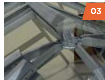
03 The aluminium rafters, ridges and wall plates are fitted and the spider arms are secured to the spider bracket.
