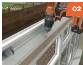
02 Timber packer and structural ring-beam are sealed and secured to the top of the window frames.
